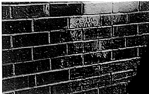
Effects of sandblasting on brick surfaces.
